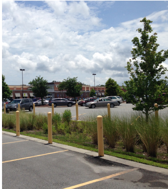
Green infrastructure elements in a parking lot.
